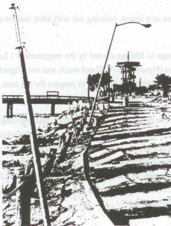
Figure V.2 Liquefaction damage, Port of Oakland
